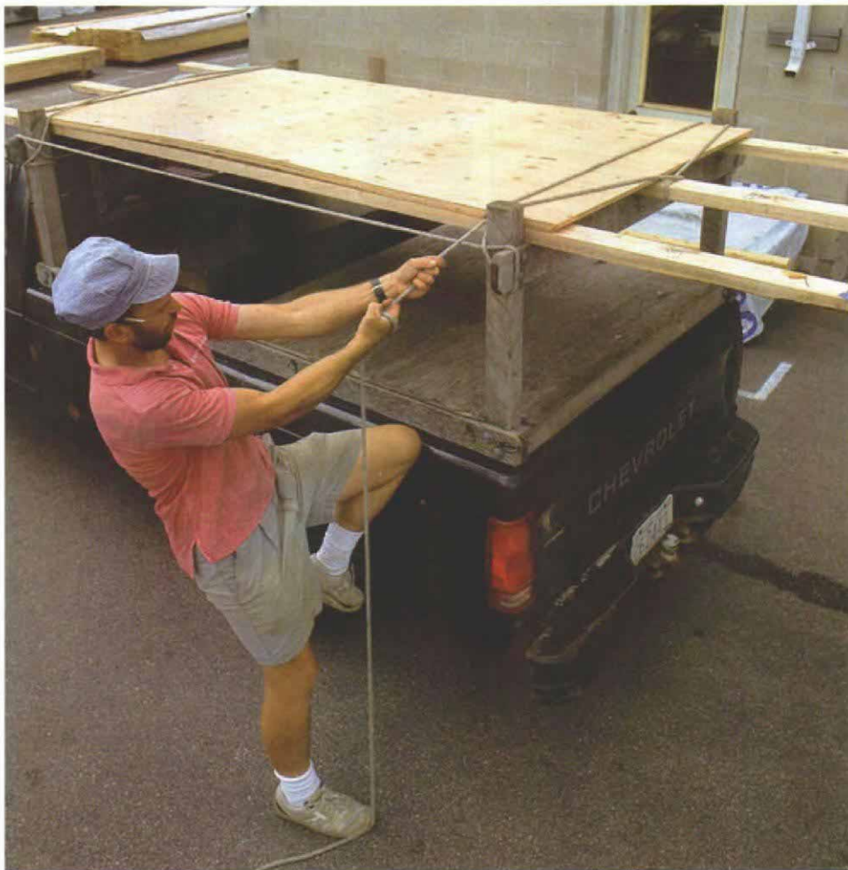
Lashing panels to a cargo rack. When transporting panel products, such as gypsum board or plywood, to the job site, the materials should be supported in the middle and restrained at the corners.
